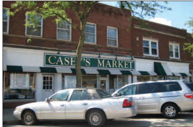
Casey's Market in Downtown Western Springs serves as an example of how façade enhancements can improve a property through fairly simple improvements. In this case, adding gooseneck lighting above the store sign and extending the awning across the entire storefront help frame the façade. Casey's Market is also a consolidation of multiple adjacent buildings, which is similar to the proposed consolidation for the 104-106 W. St. Charles Road properties in Downtown Lombard (see Figure 3.3 for façade enhancements for the consolidated building).
