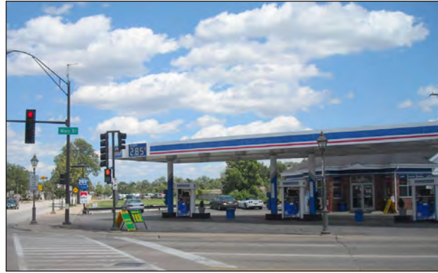
Reducing driveway widths is one method to help minimize curb cuts along roadway corridors; for example, the driveways serving the Marathon gas station could be reduced.
