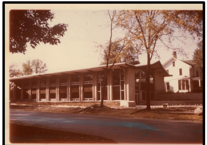
Figure 4 Historic view prior to Plum House being demolished, courtesy of Lombard Historical Society
