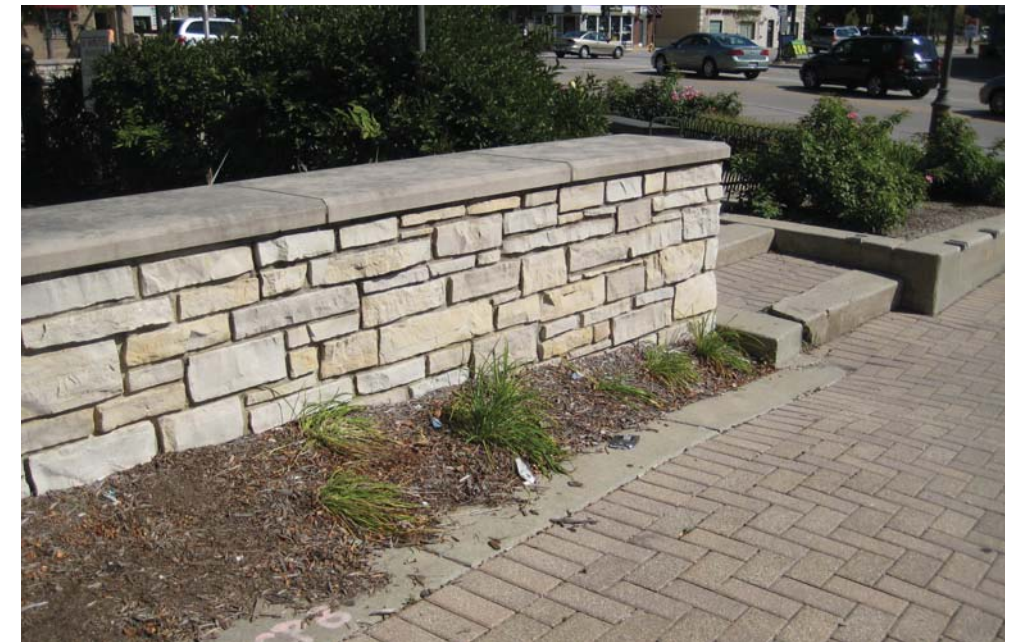
Limestone Wall with Precast Cap
